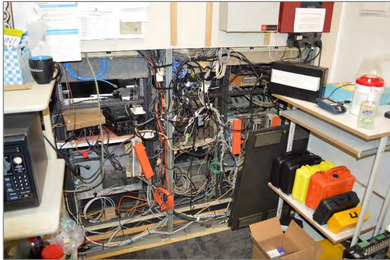
Former Dispatch Room
