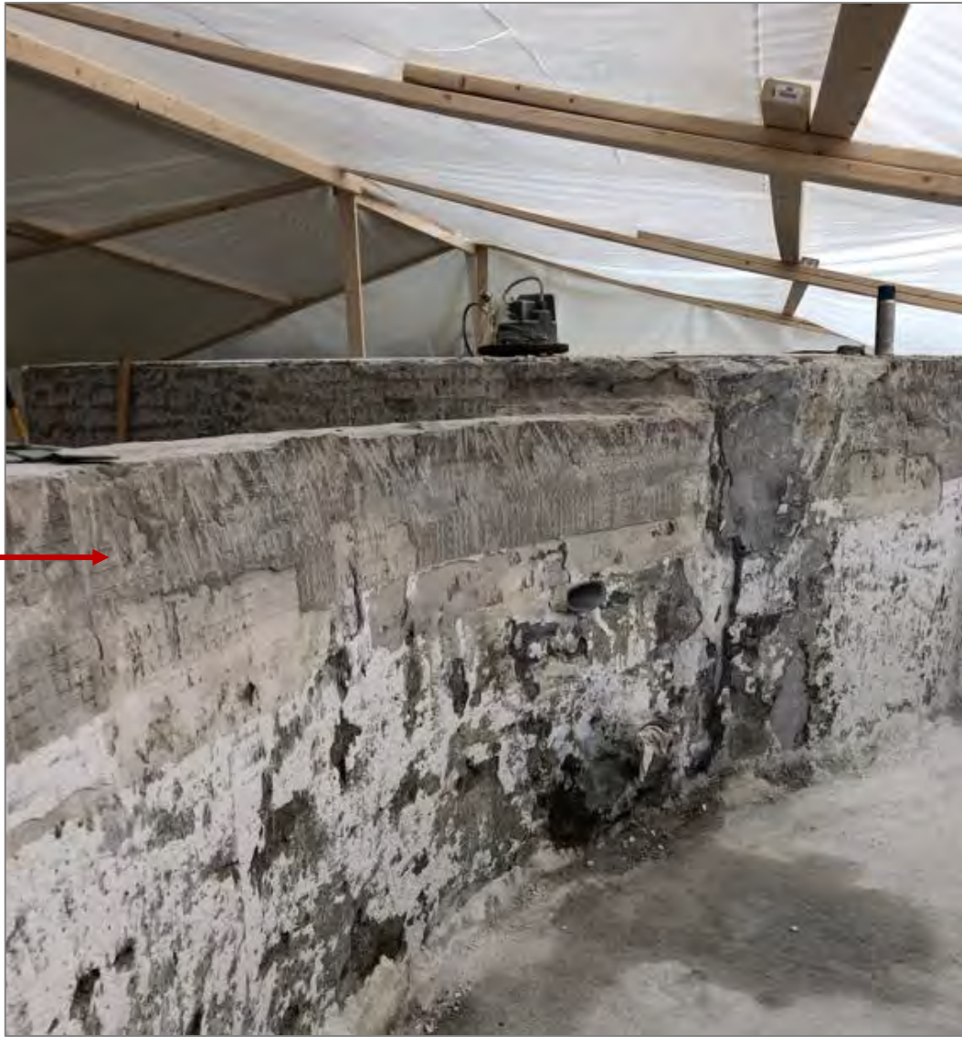
Leisure pool finish removed to expose moist, deteriorated concrete
